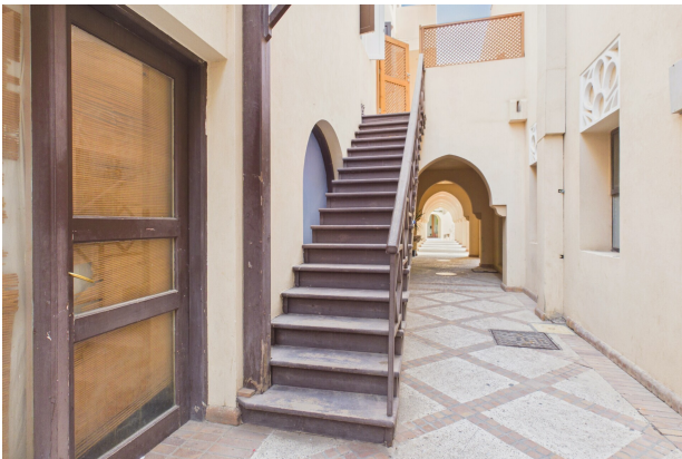
Stairs to Terrace
